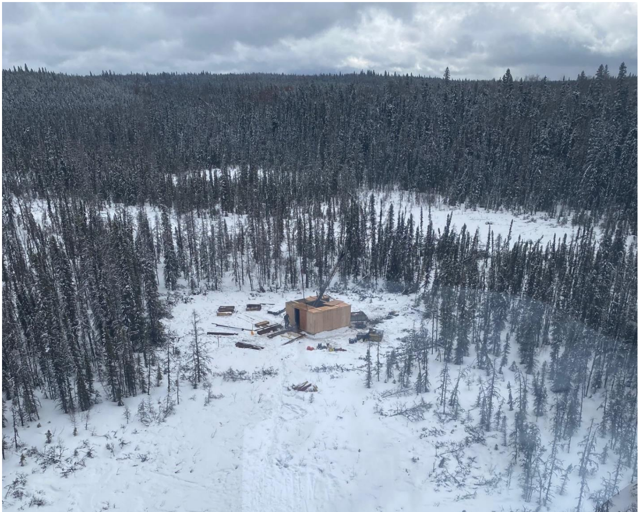
Figure 1 - March 23, 2022, photograph taken by Jake Ziehlke aboard Gogal Air Services helicopter as daytime drill crew arrives on-site to continue drilling operations at the Zoro Project in Snow Lake, Manitoba.
