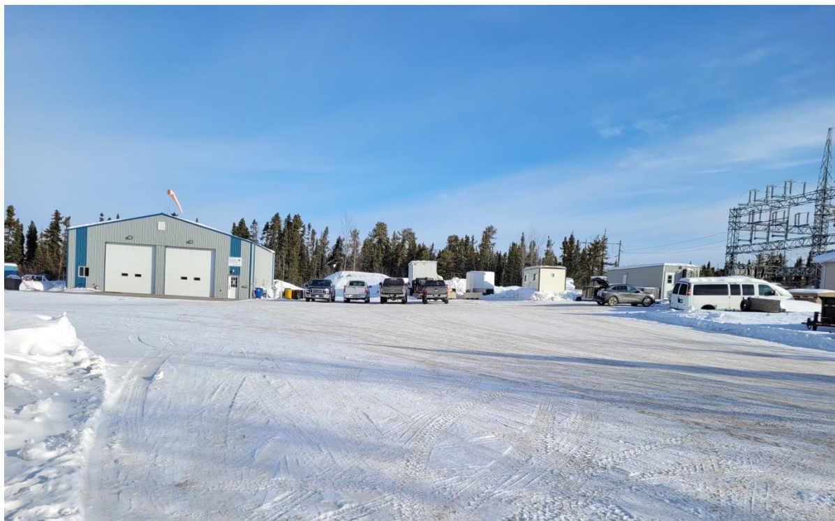
Figure 2 - picture of Gogal Air Services set-up for core logging and logistical command center.
