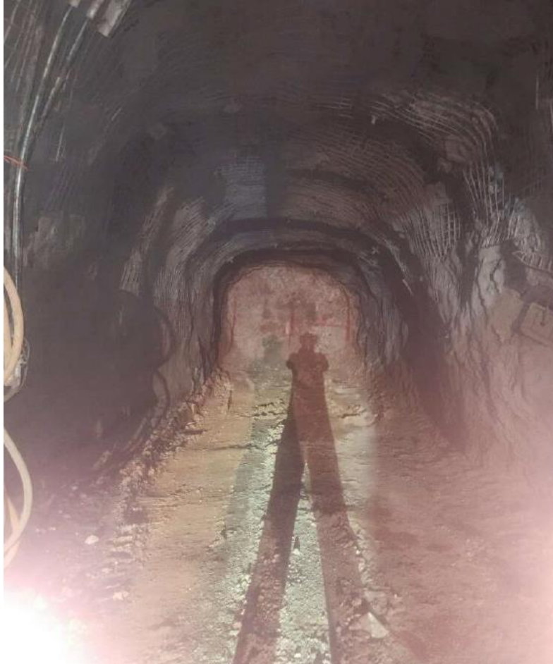
Shotcreting and rock bolting has been extended to depth
