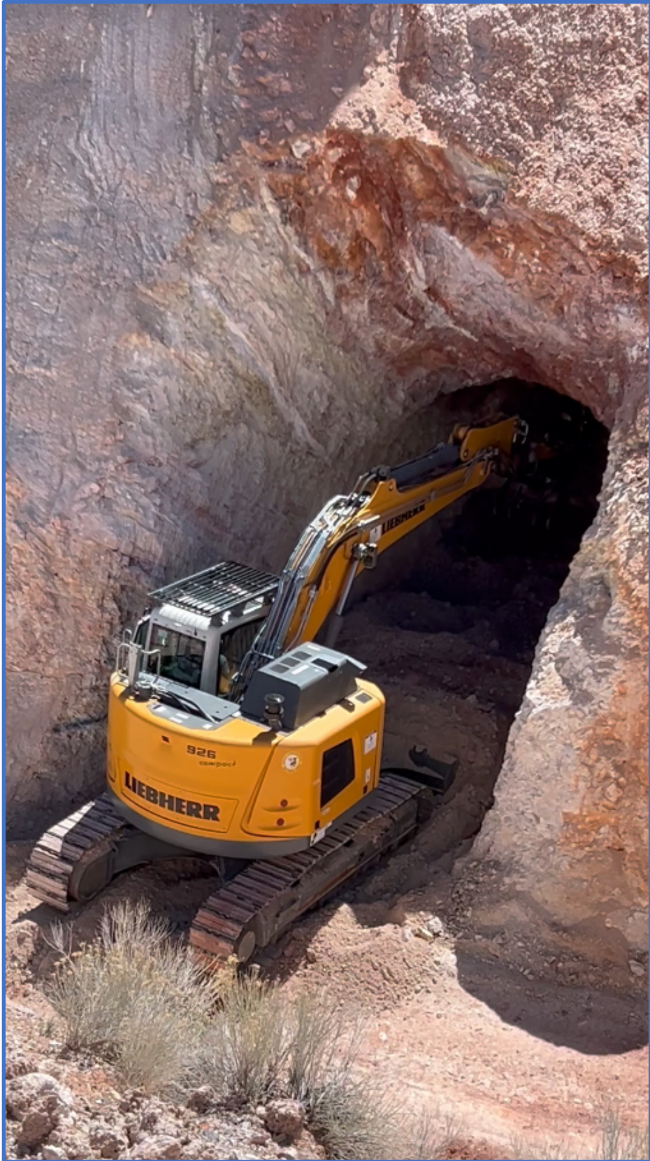
Figure. 1 - Ramp installation begins at Ares' Fluorspar Mine
