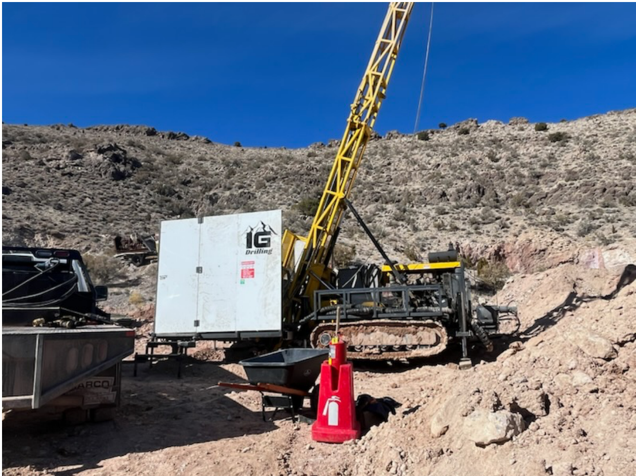
Delineation Drilling Begins at Mine Site
