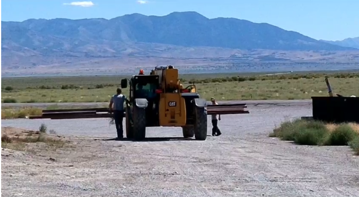
Moving and Positioning Steel Structures
