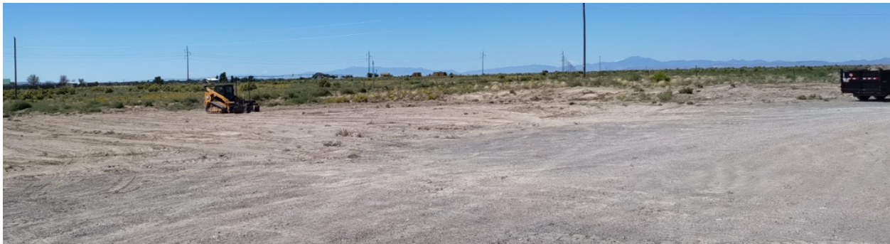
Clearing and Levelling Plant Site
