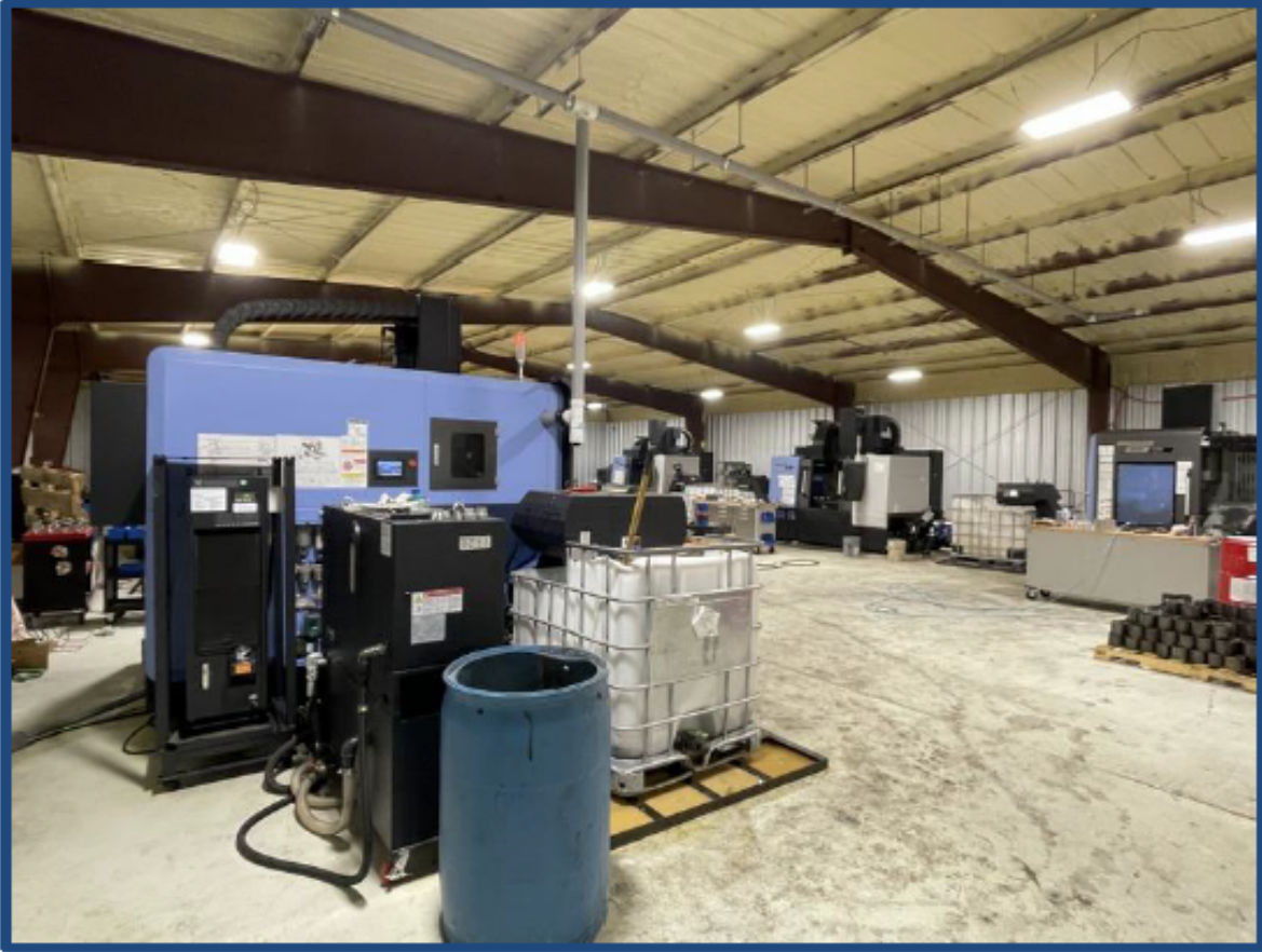
New Facility and Warehouse Installation
