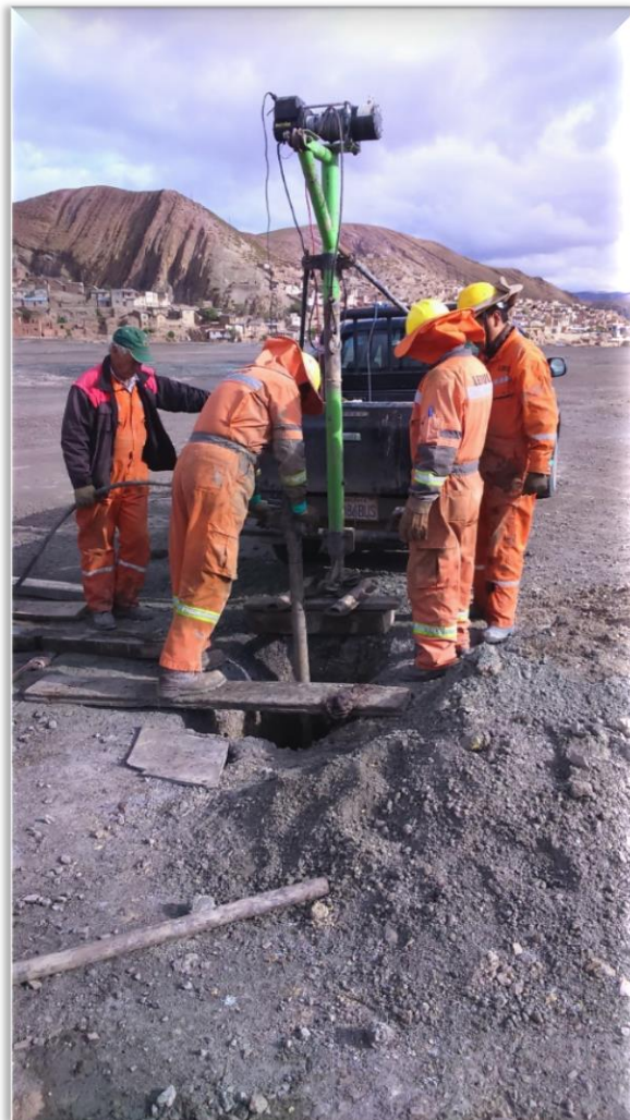
PICTURE 10.1 VIBRACORE DRILLING EQUIPMENT
