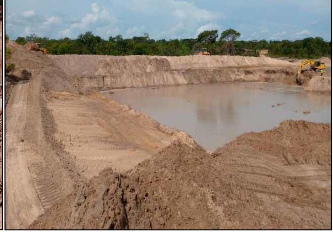
Fig.2 Tailings storage Facility excavation
