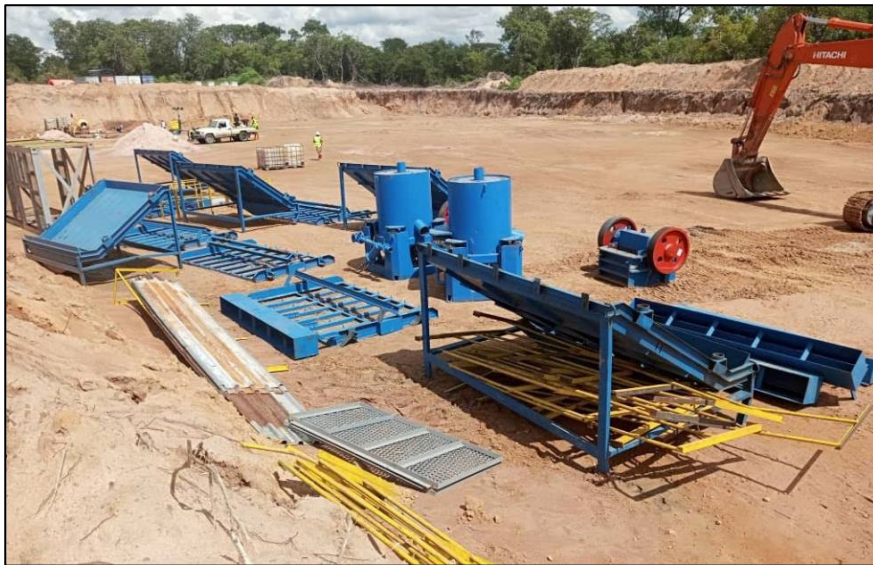
Fig.3 Equipment arriving at Project Site
