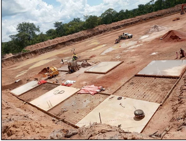
Fig.1 Concrete works for Plant Equipment
