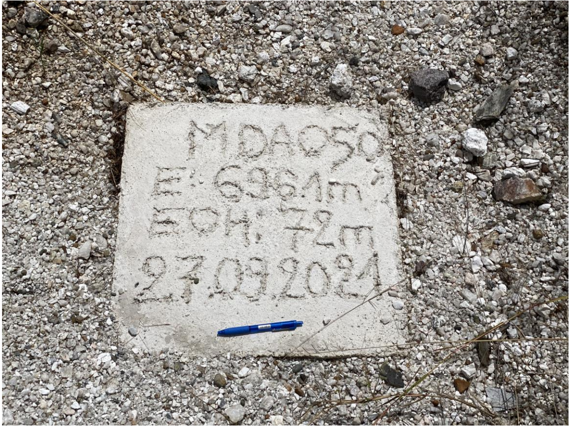
Figure 10-4 Concrete plinth over collar MDA050
