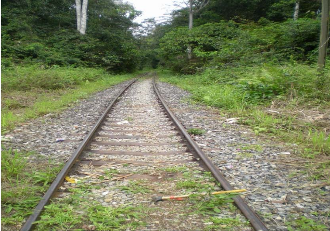
Picture 4: A view of the Camilog “Cape Gauge” narrow gauge railway. Note the steel sleepers dating from 1976 and the approximately 70 lb/yard rails, inadequate for the anticipated transport of iron ore.
