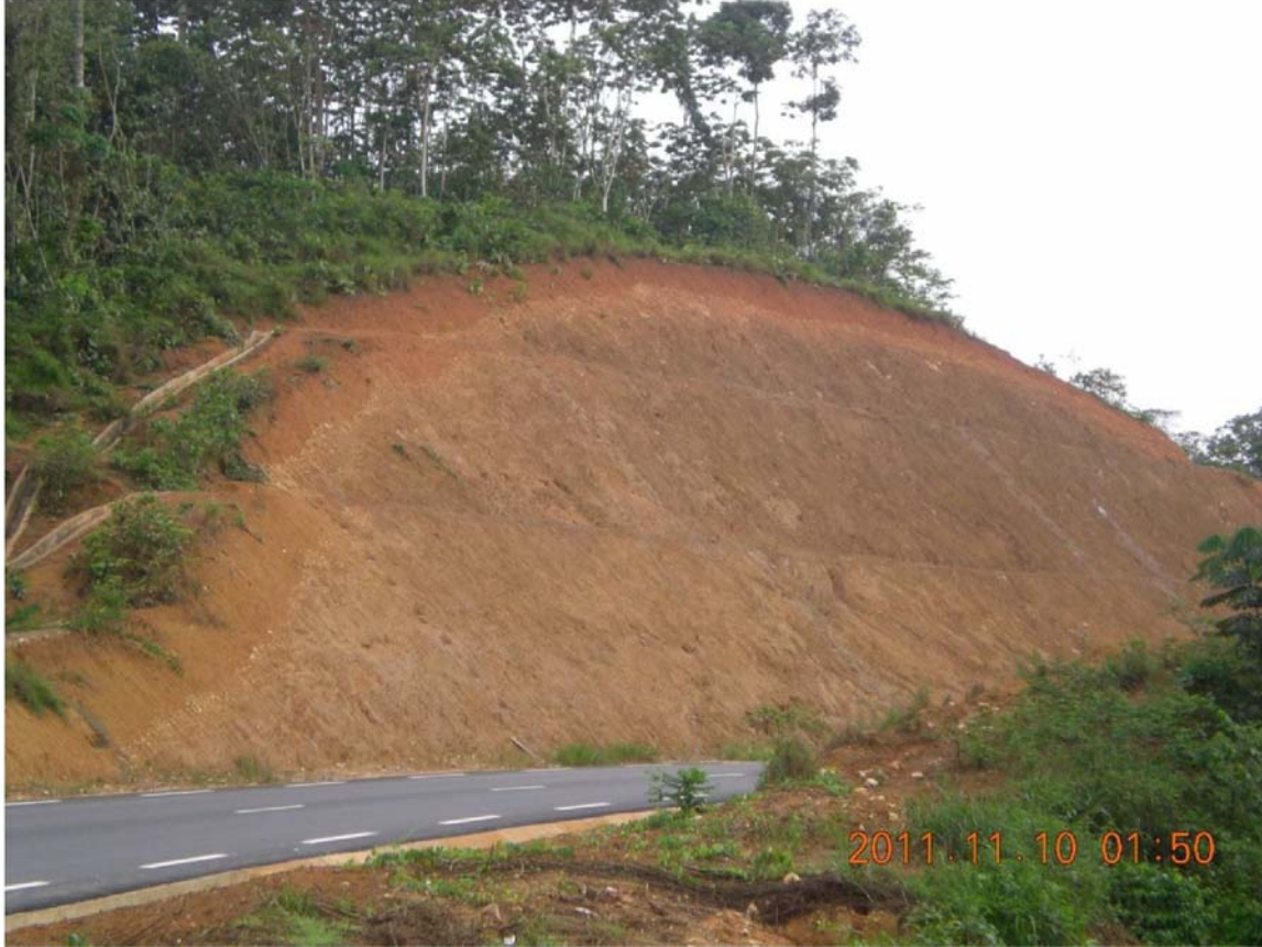
Picture 9: A view of a road cut along the Pointe-Noire - Brazzaville N-1 highway through the Mayombe mountain range. The bedrock is a completely laterized schist or gneiss. Note the 1-2 meter thick zone of bioturbation at the surface (ochre layer) and the underlying laterite, where the mud has preserved the ghost structures of the original rock (foliation dips to the right).
