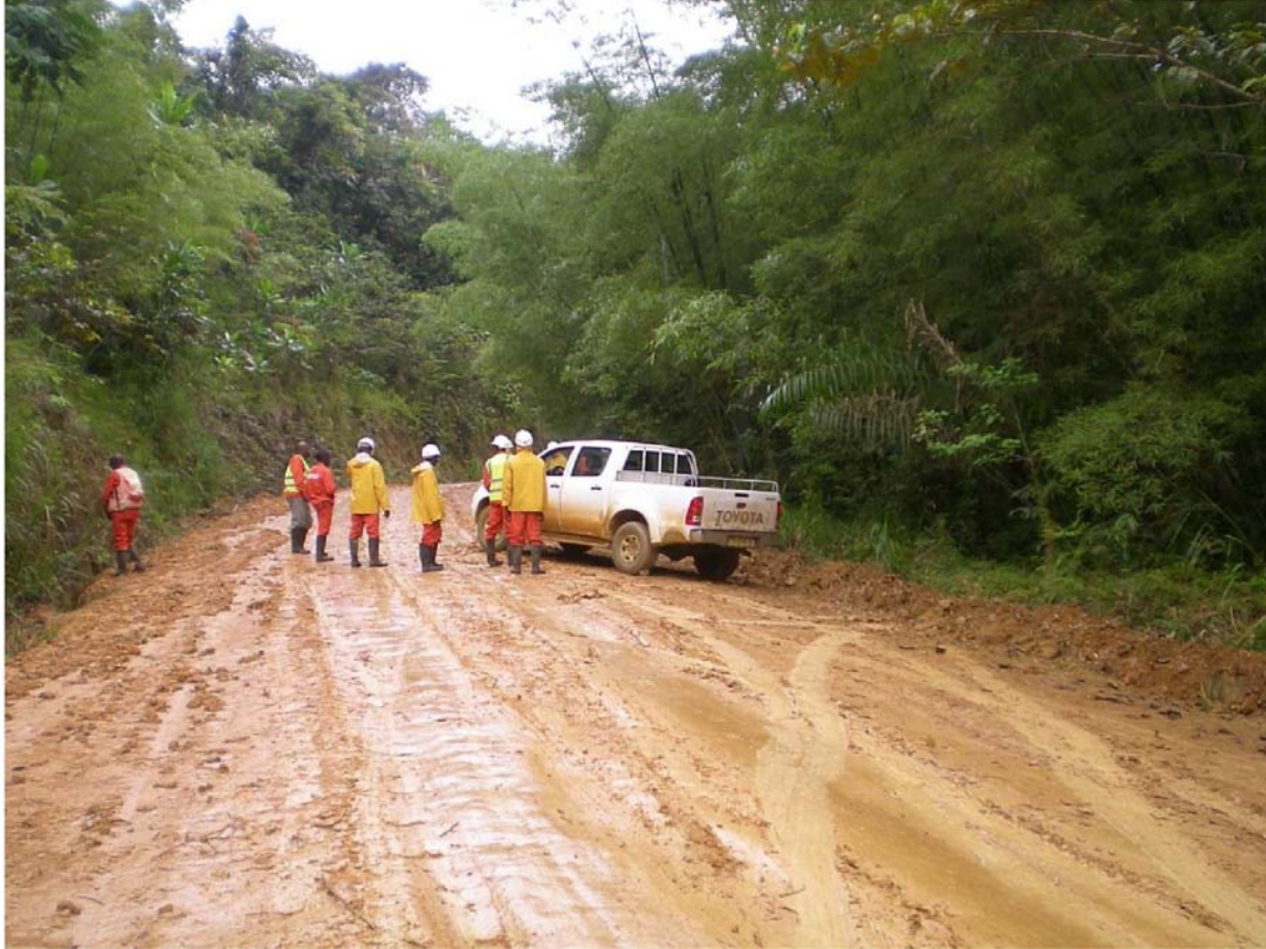
Picture 3: View of N2 national road leading to Mayoko. Notice that the lightest rain renders this mud track extremely slippery and near impassible. The 4x4 pickup in the picture was immobilized by a 1-2% grade hill!!
