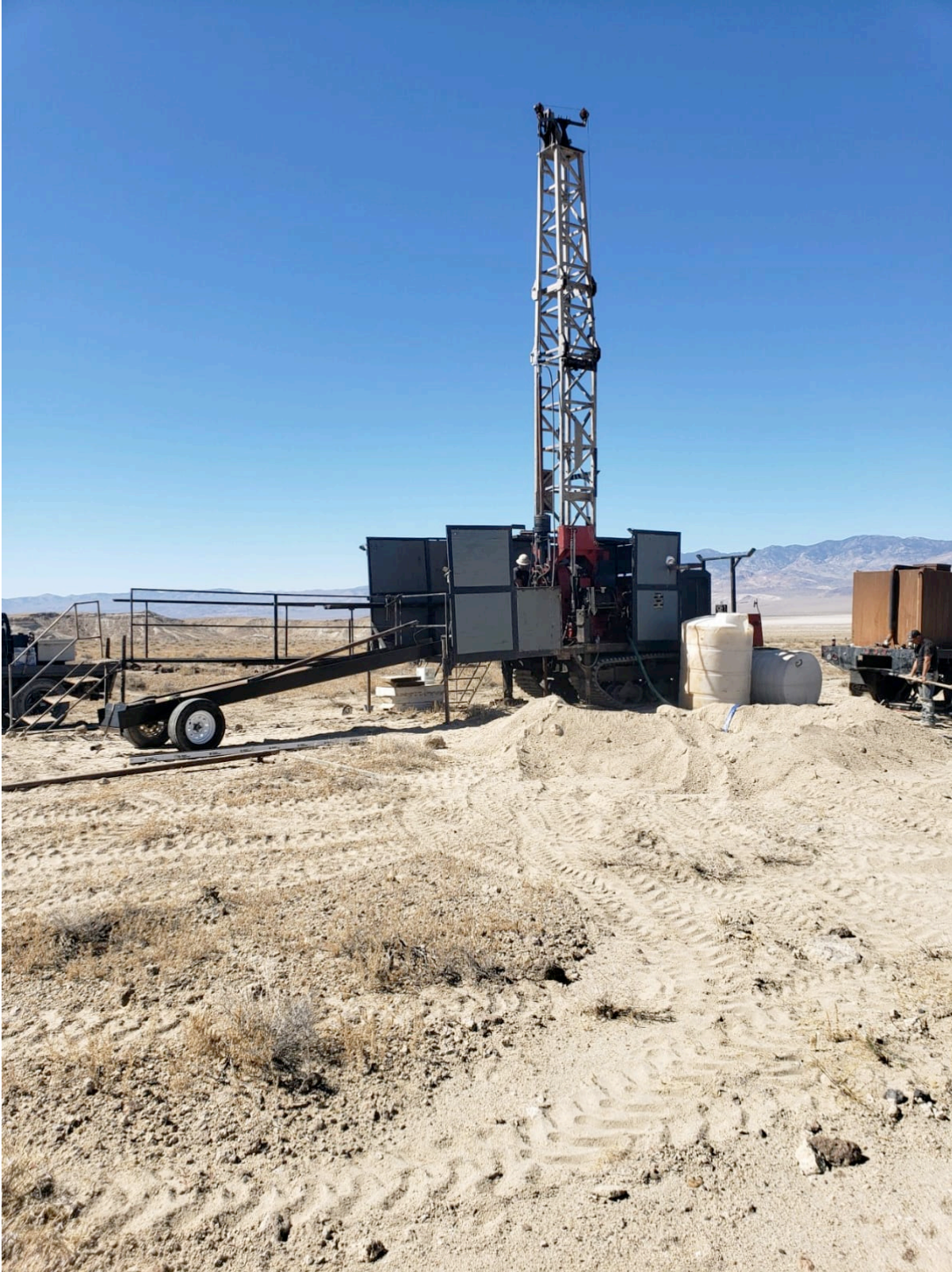
*Clayton Valley drill rig on site
