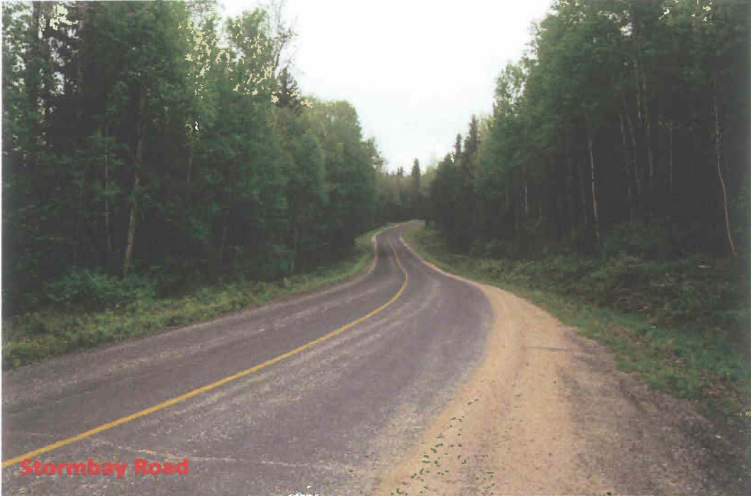
Figure 4.3 Photos showing the general condition of roads used to access the Black Jack Project area.
