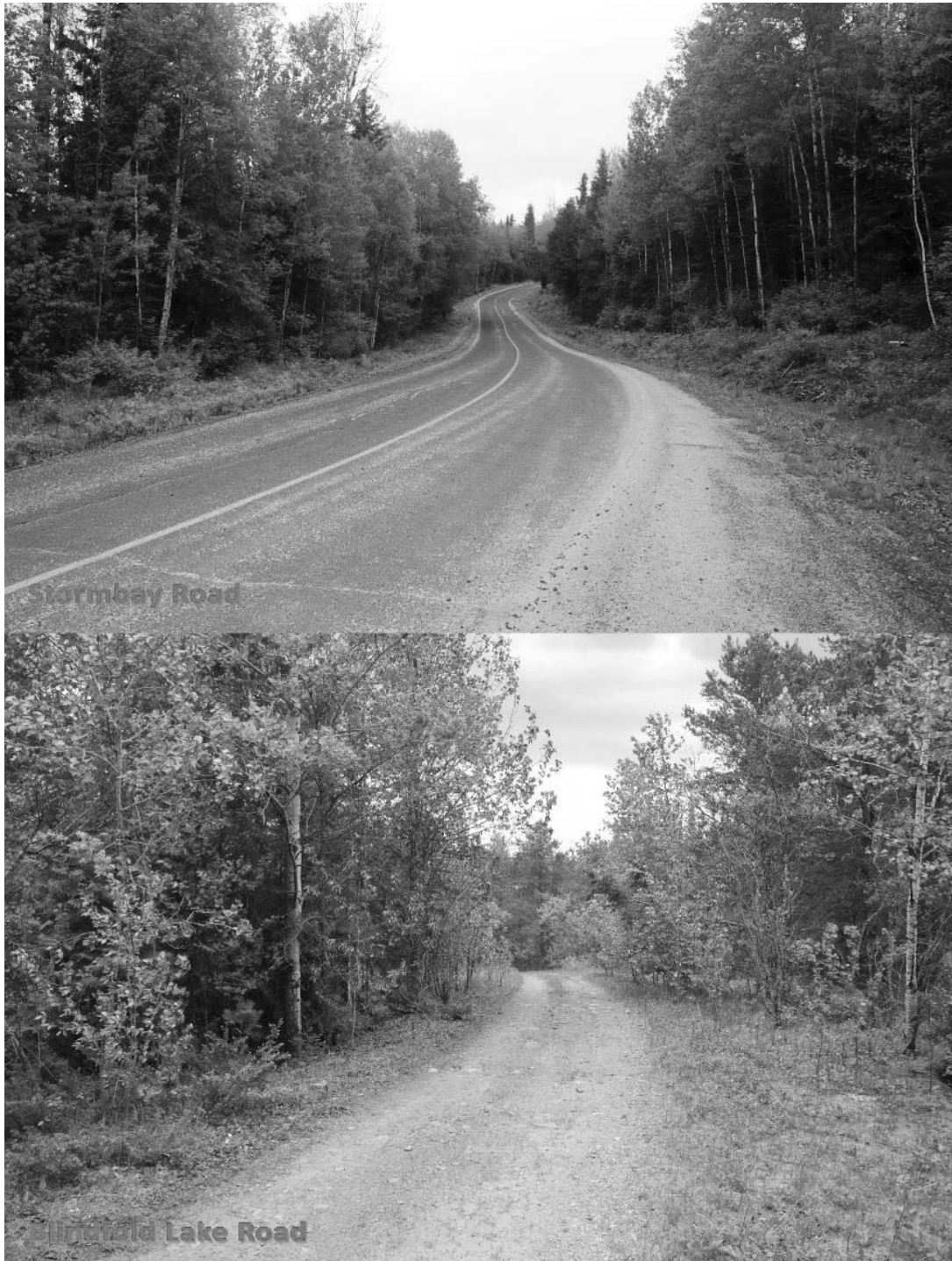
Figure 5-1 Photos showing the general condition of roads used to access the Black Jack Project area.
