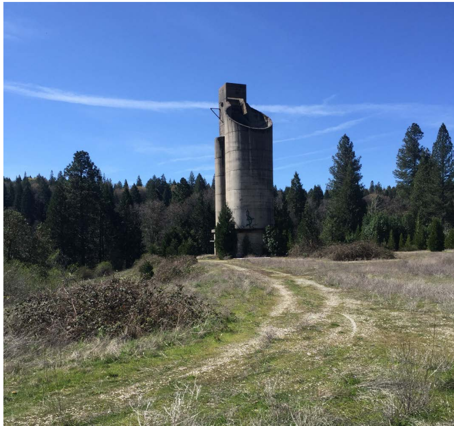
Figure 12-1: Concrete Rock Silo Adjacent the Brunswick Shaft; View Looking West
