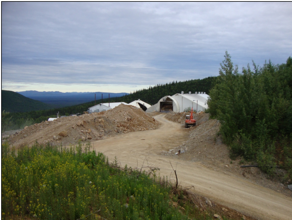
Figure 4: High Grade Stockpile (left) and Medium Grade Stockpile (right) ahead of Primary Crusher
