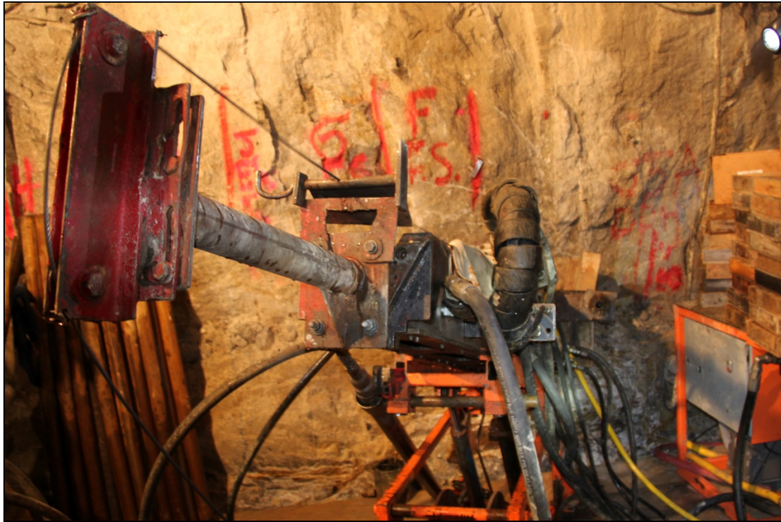
Figure 7: Hagby Drill Set Up Underground
