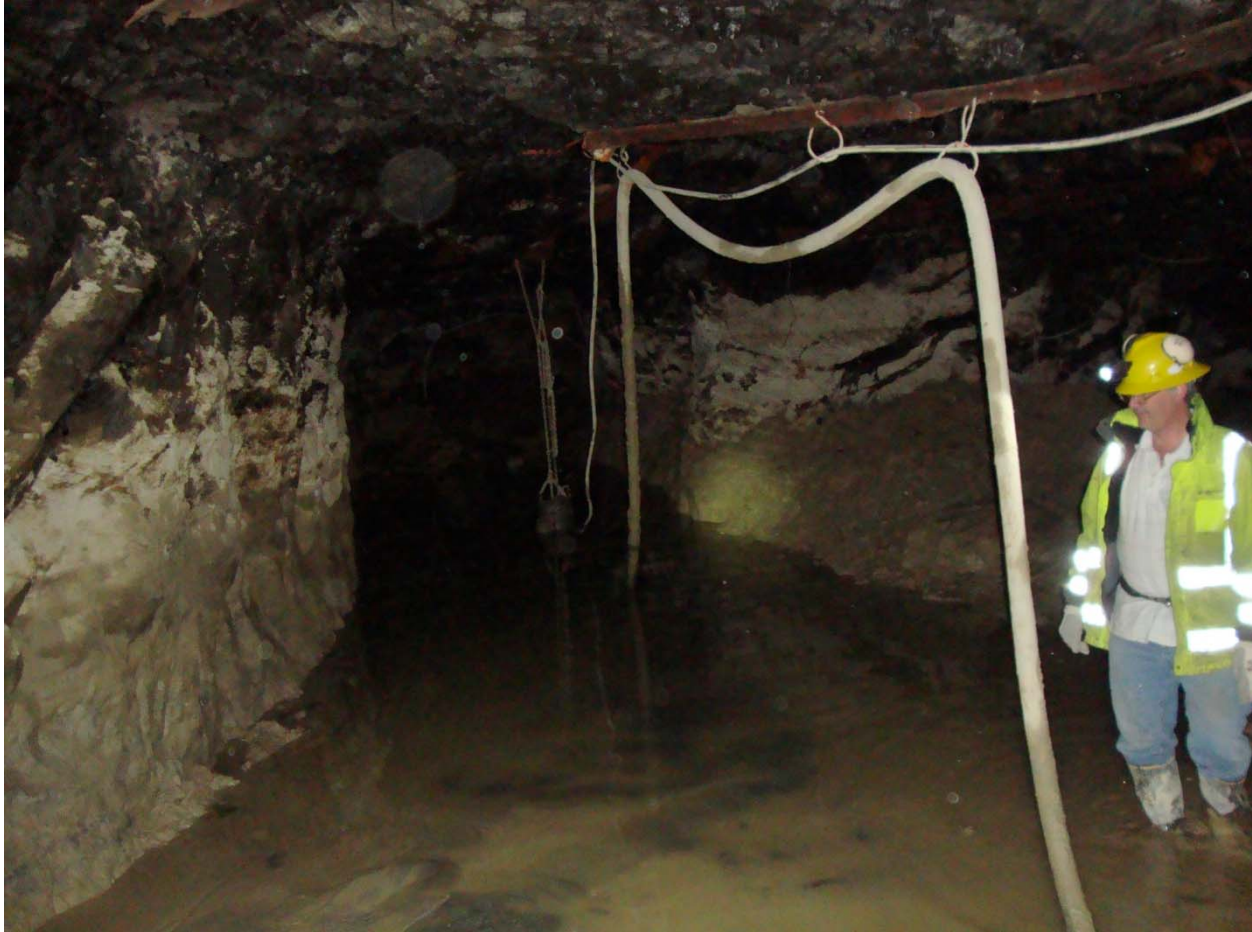
Figure 7: Old Ramp Bottom
