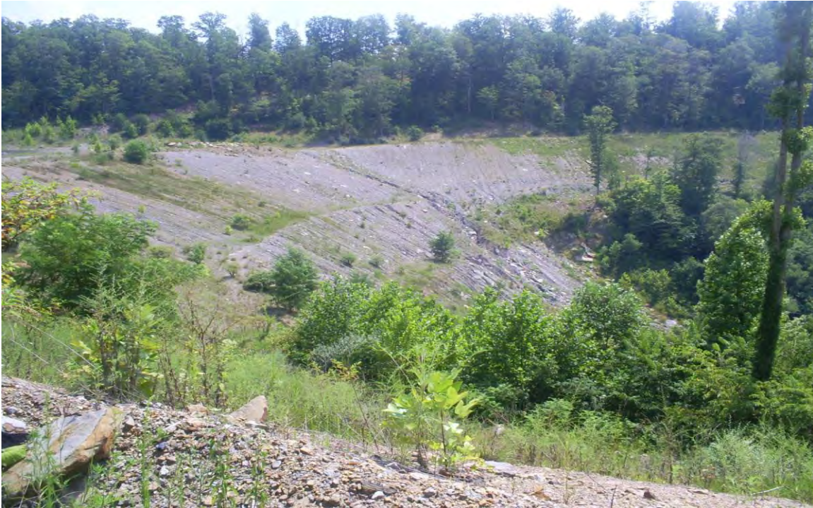
Existing excess spoil fill constructed by Minnehan Mining, LLC.
