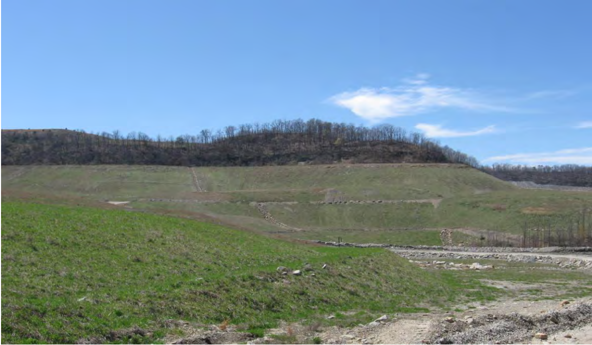
Reclaimed areas near entrance of permit.
