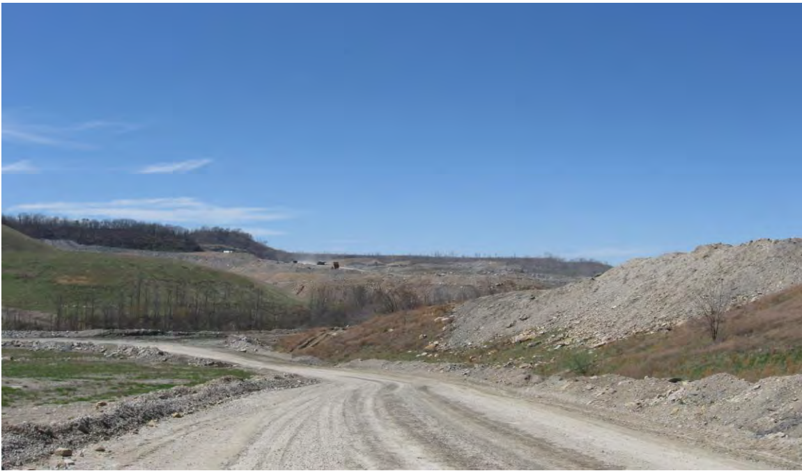
Entrance Road: Cheyenne Resources permit.
