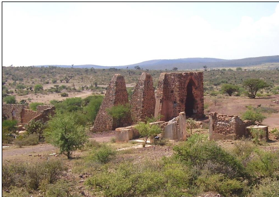
Figure 6-1 Main Shaft at the Bilbao Project
