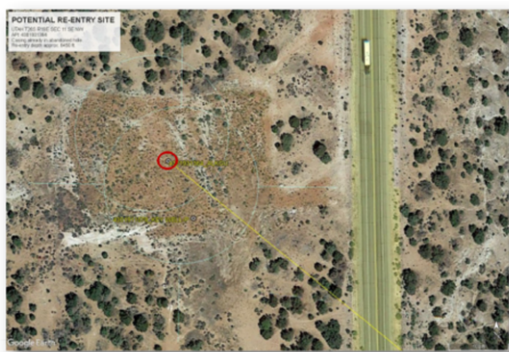
Figure 10.18 - Google Earth Image for Aviara Energy Corporation Cane Creek Federal # 11-1 drill site.
