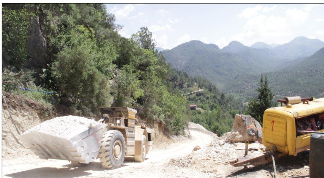
Figure 5: Pinargozu mine portal access road Showing typical mountainous terrain with extensive tree cover
