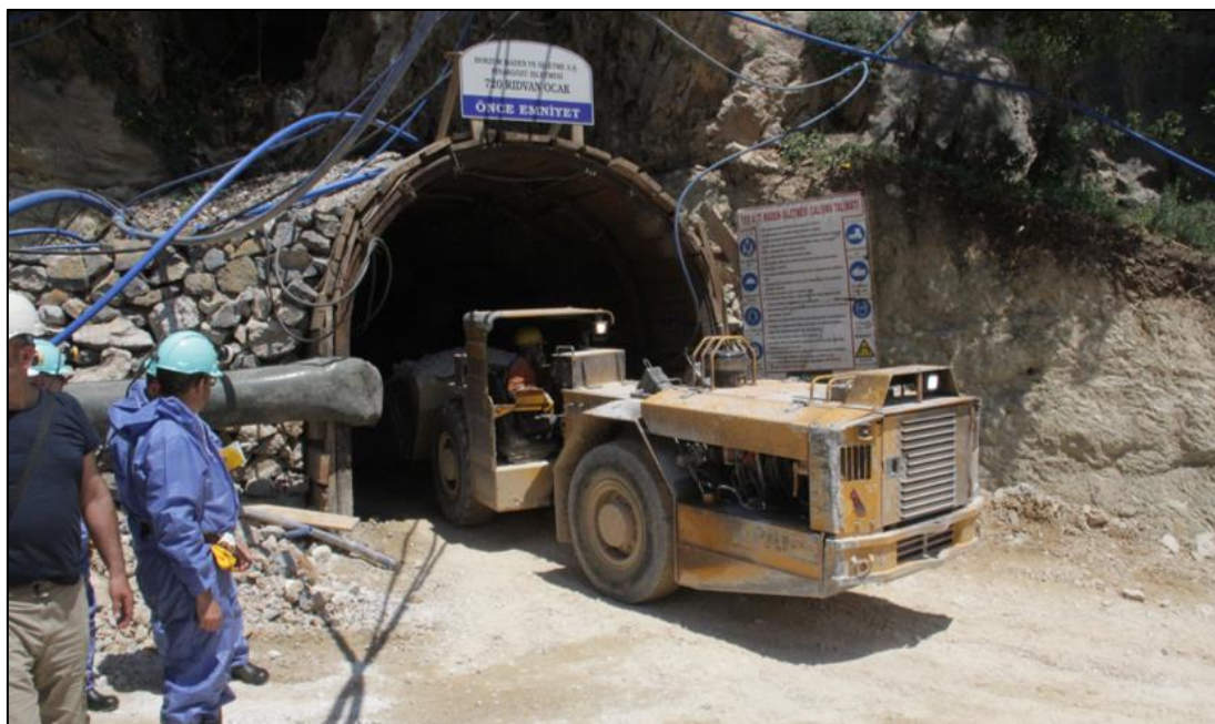
Figure 4: Pinargozu underground mine adit portal
