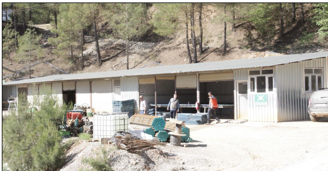
Figure 42: Core handling, sampling and preparation facility at Horzum
