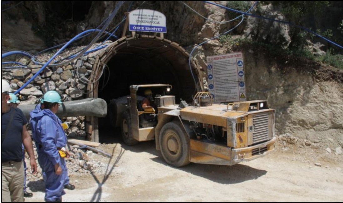
Figure 4: Pinargozu underground mine adit portal
