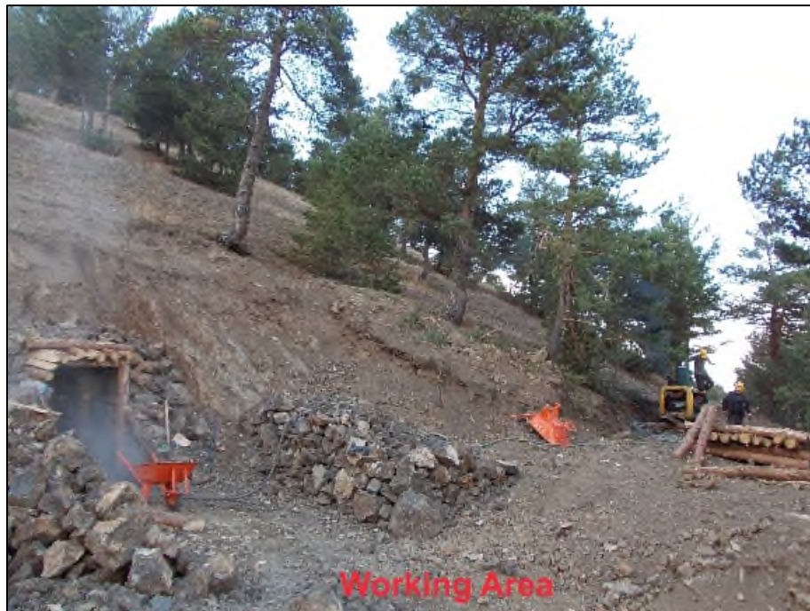
Figure 33: Photograph of 2012 adit portal.
