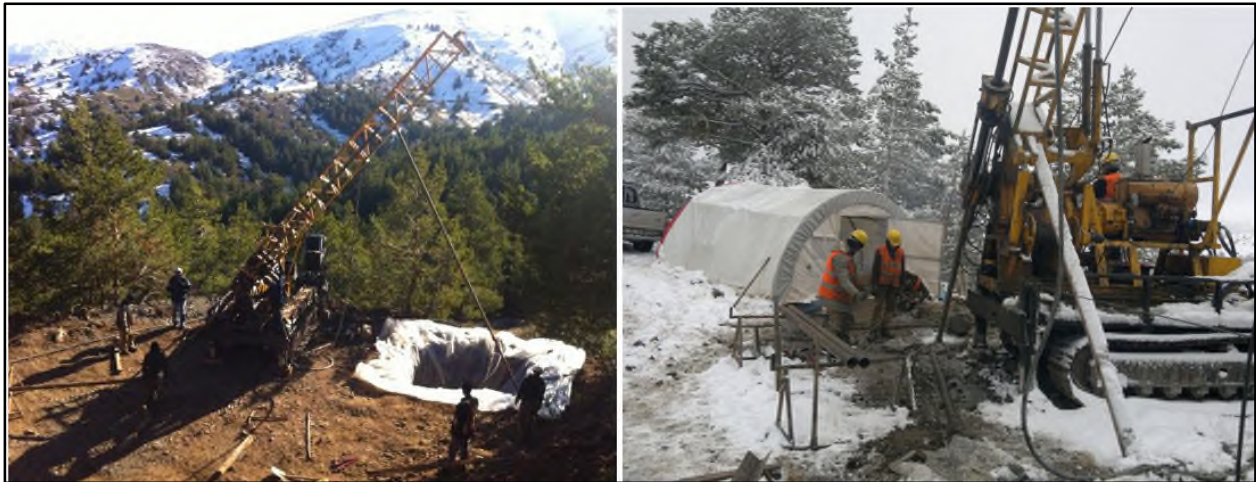
Figure 39: Pasinex drilling operations at Golcuk.
