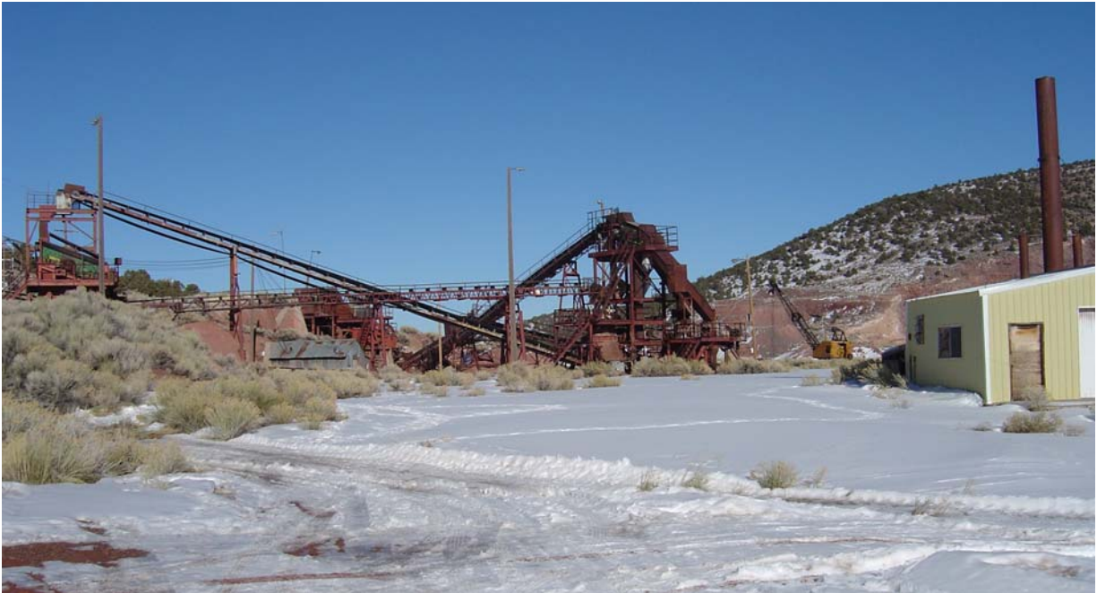
Figure 6.1 Atlanta Mill - Crusher Complex
