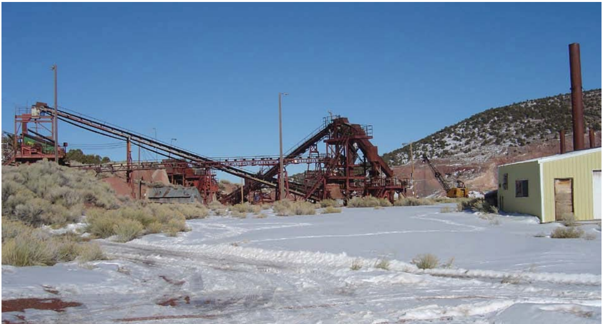
Figure 6.1 Atlanta Mill - Crusher Complex
