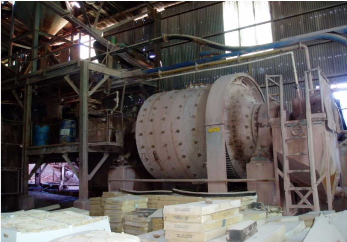
Figure 6.2 Atlanta Mill – Primary Ball Mill
