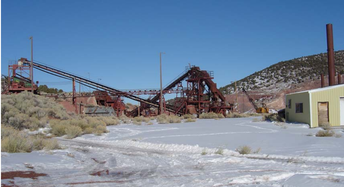
Figure 6.1 Atlanta Mill - Crusher Complex
