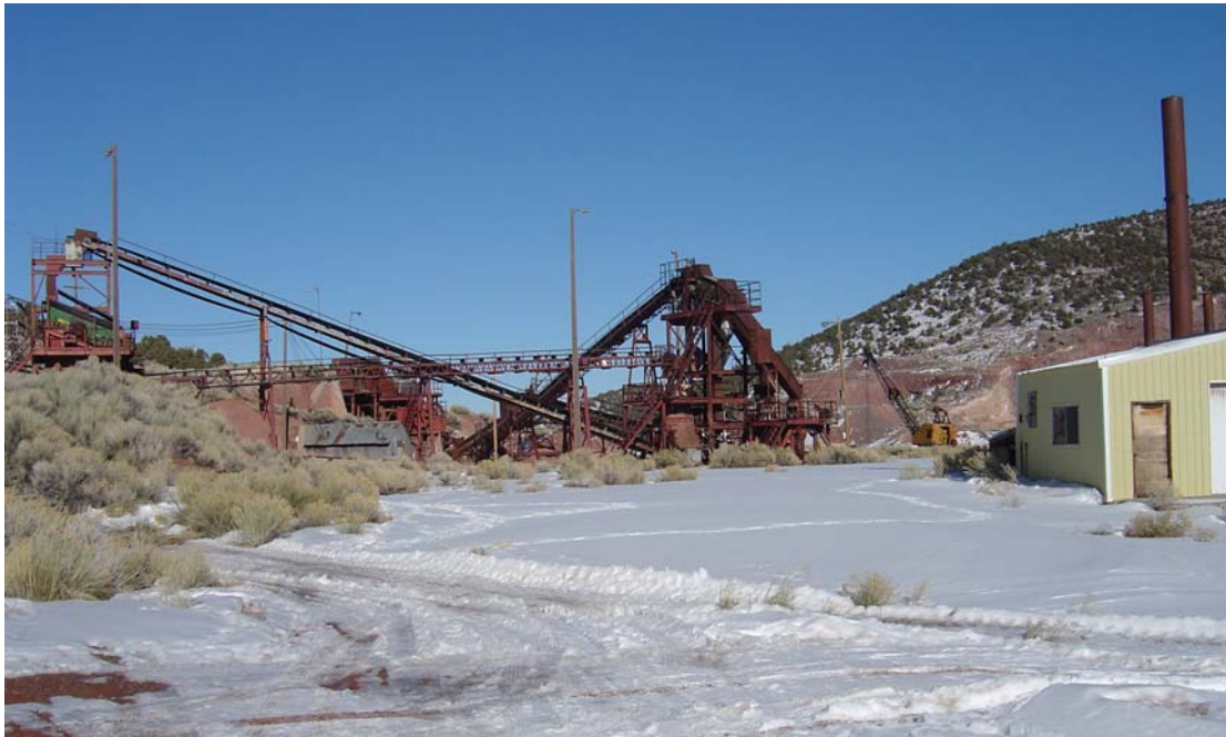
Figure 6.1 Atlanta Mill - Crusher Complex
