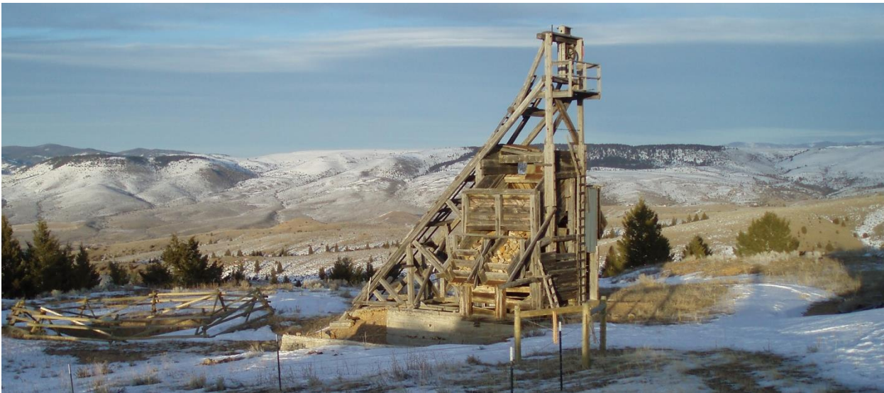
The headframe of the St. Lawrence mine inclined shaft
