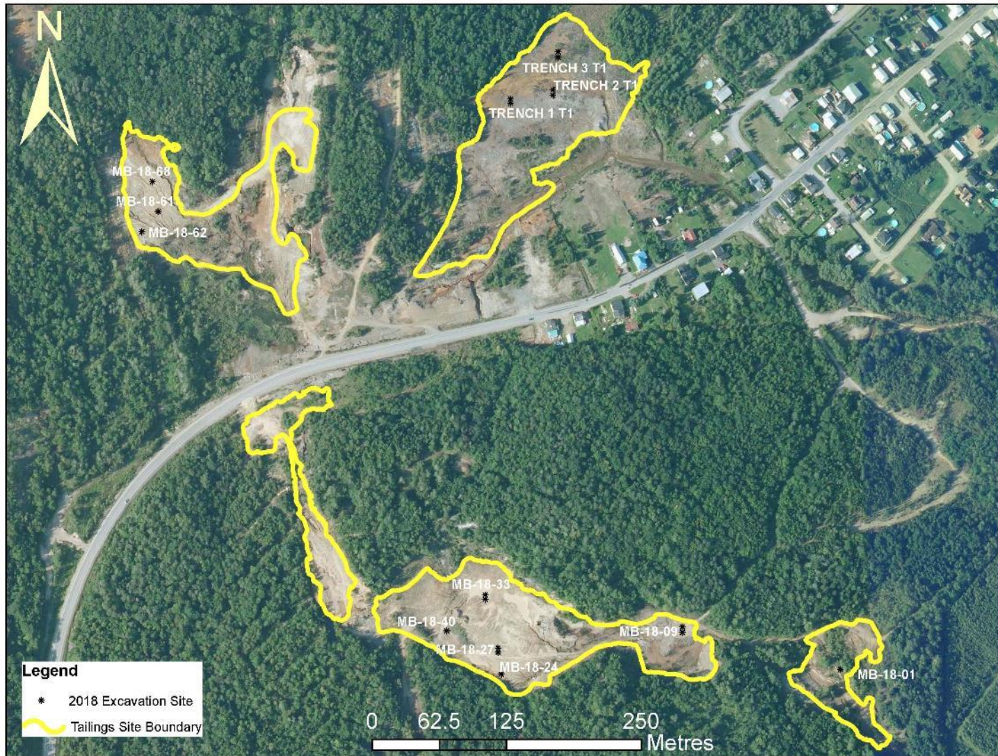
Figure 6.4: Locations of 2018 trench/pit excavations by 1844 Inc
