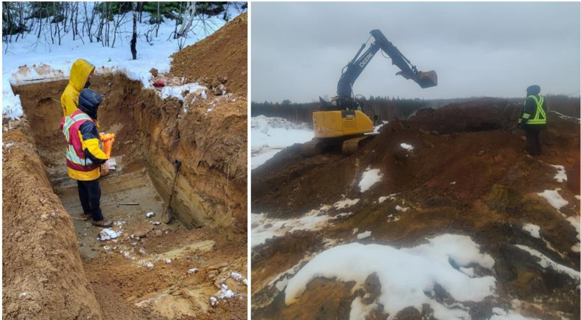
Figure 9.3: Typical test pit excavations
