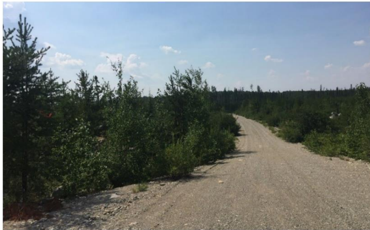
Figure 5-1: Eagle River Property Access Road Used During 2020 Site Visit
