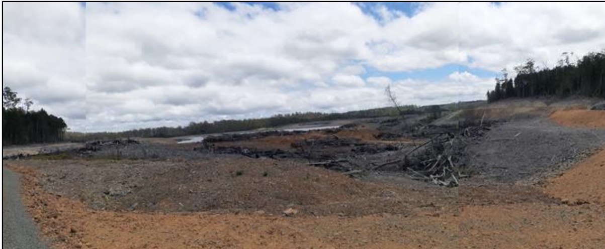
Figure 18-3. Hellyer TSF2 under construction, showing significant timber waste vegetation material
