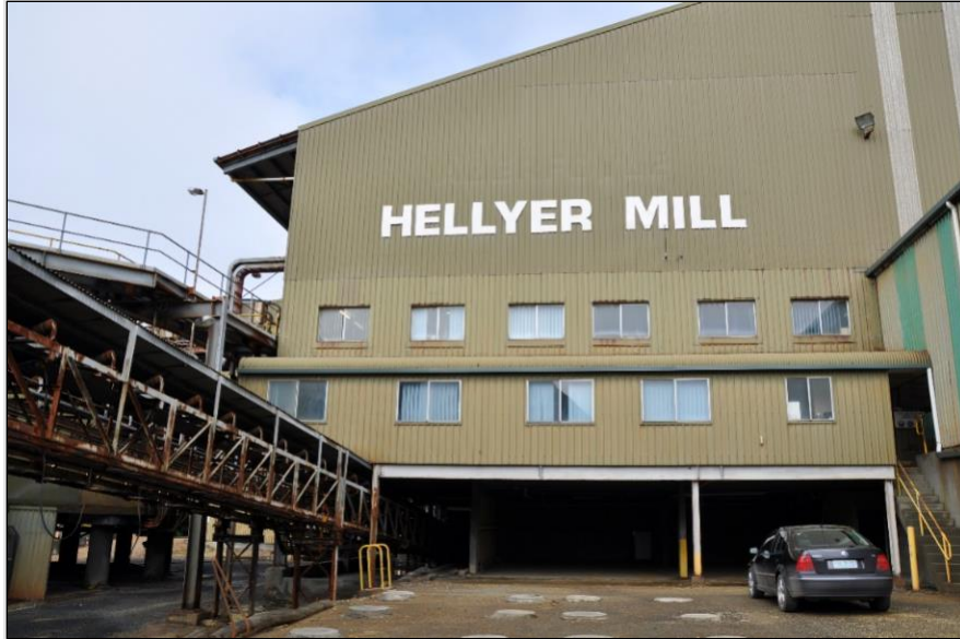
Figure 18-5. View of Hellyer Mill from outside
