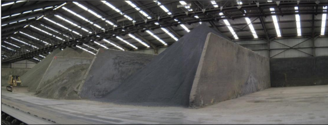
Figure 18-7. View of the concentrate shed from inside at the Bernie Port.
