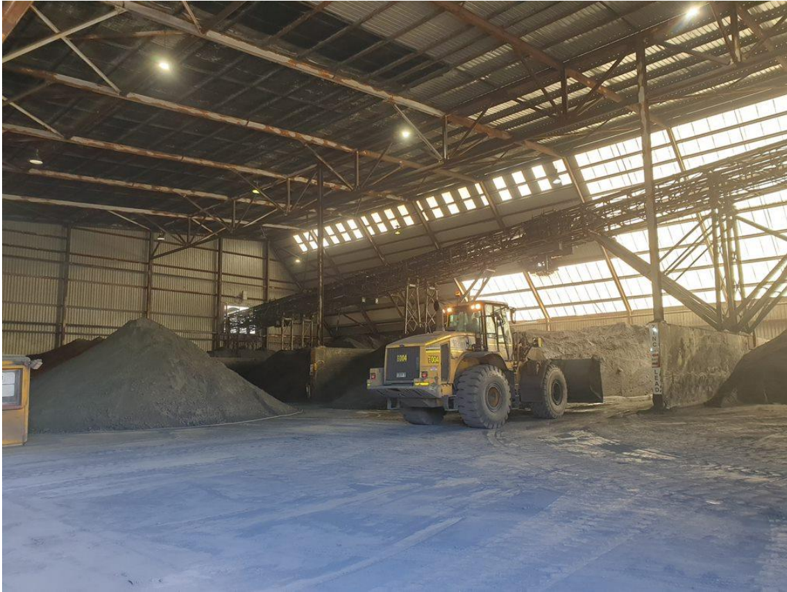
Figure 7-3. Concentrate load out shed at the Hellyer Gold Mine
