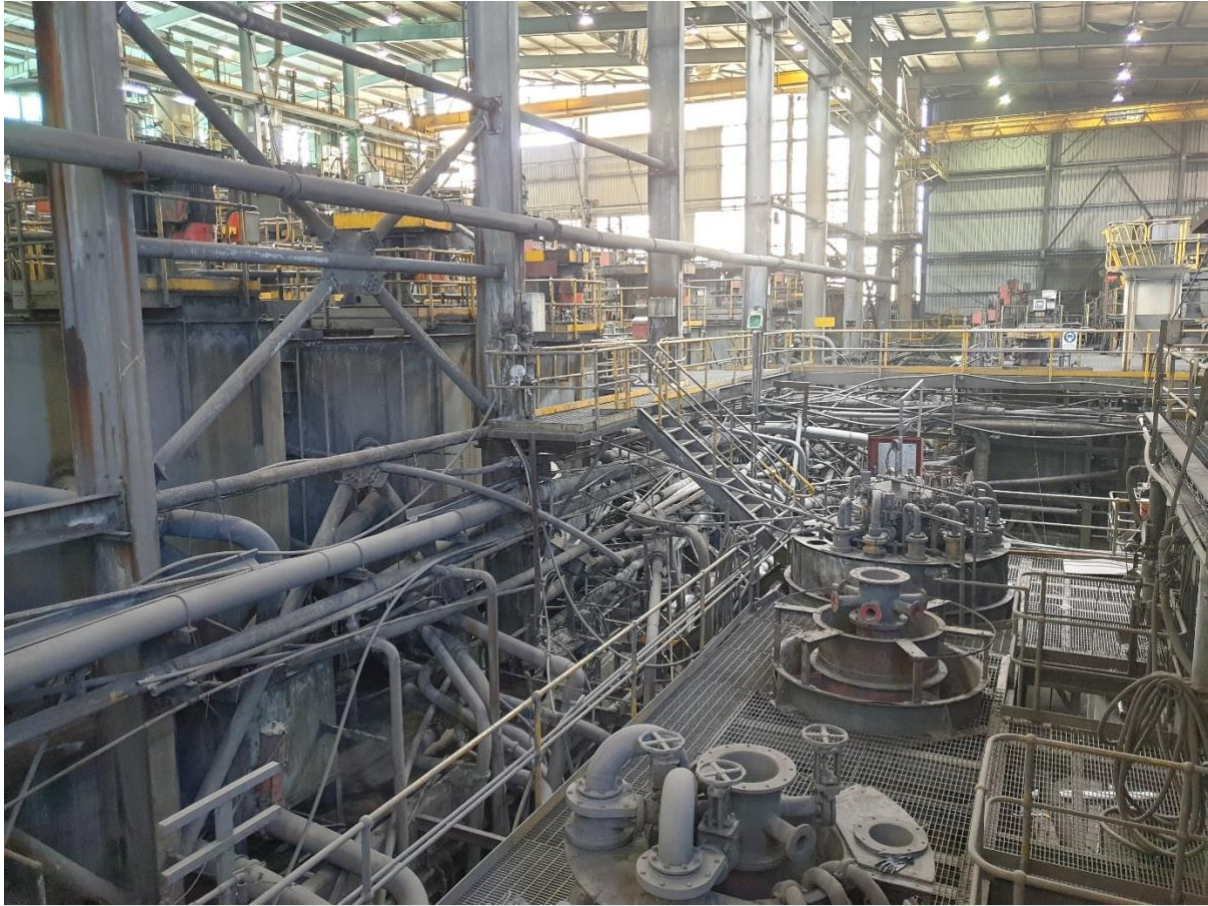
Figure 7-4. Hellyer Processing Plant General View
