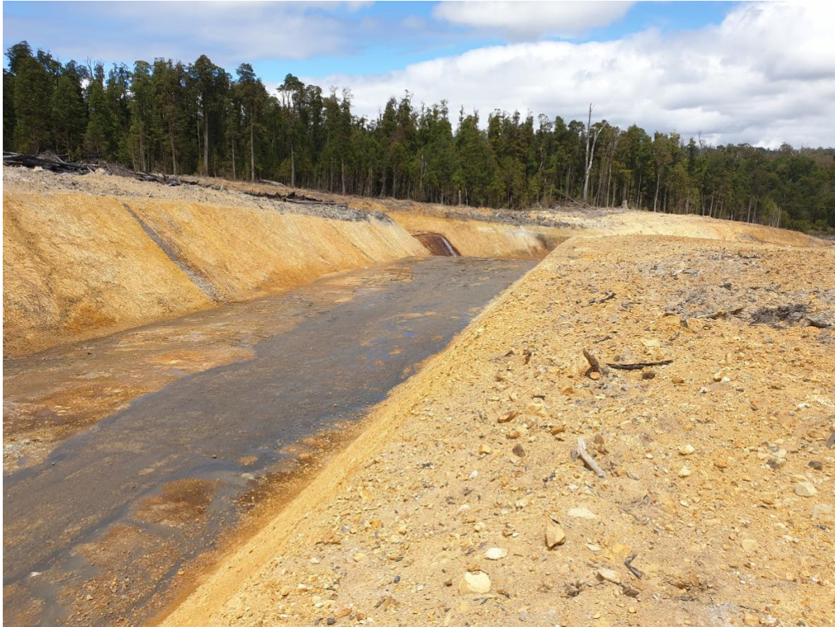
Figure 6-2. Emergency spillway at the tailings storage facility for Hellyer Gold Mines
