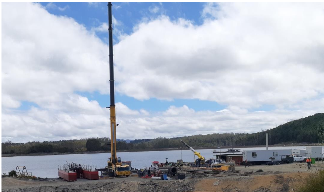
Figure 16-2. Beaver 40’ dredge, being constructed at Hellyer TSF1
