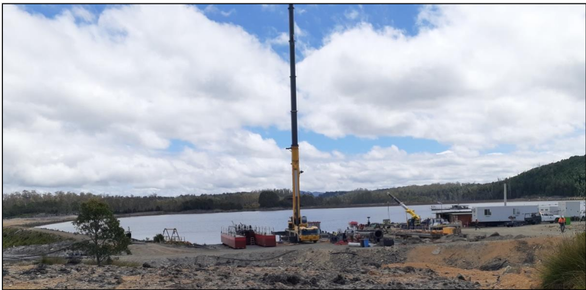
Figure 7-5. Hellyer Tailings Storage Facility (TSF1) showing new “Beaver” Dredge commissioning site
