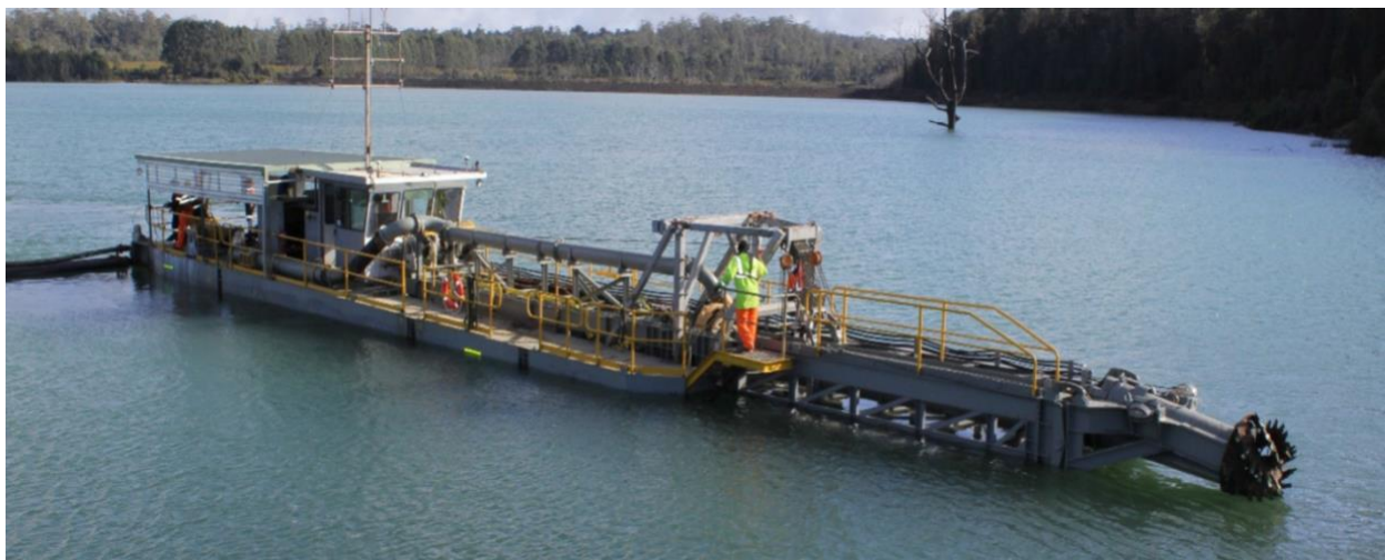
Figure 16-1. Seabird III dredge on Hellyer Tailings Dam
