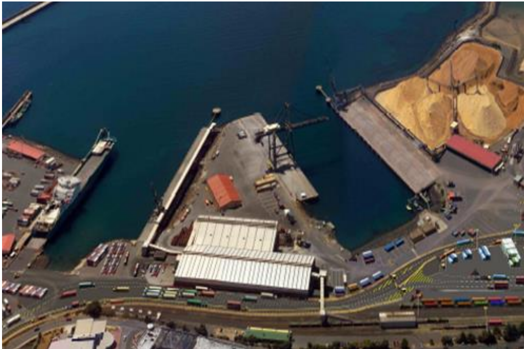
Figure 18-4. View of concentrate shipment facility in Burnie
