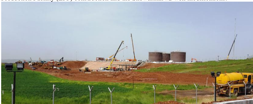
Shewashan EPF under construction – April 2017
