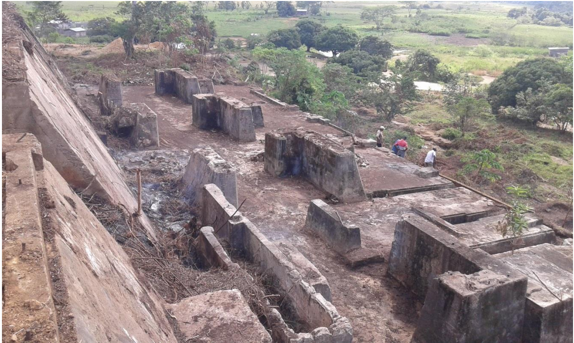
Photo 17.3 Photograph of existing old plant area – after clean-up (DENM 2016)
