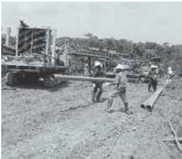
Drilling at Kaniago, March 2011.
