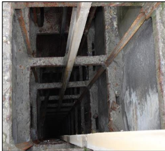
Figure 6.5: Looking down the two compartment Santander Shaft. Source CDPR (2021).
