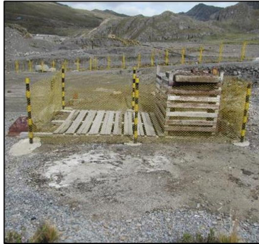
Figure 6.4: The Santander Shaft at Surface. Source CDPR (2021).
