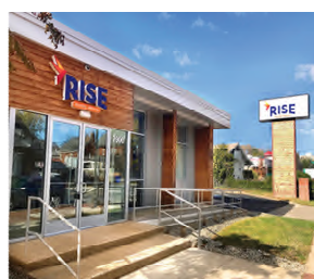
EXTERIOR OF RISE SILVER SPRING Silver Spring, Maryland
