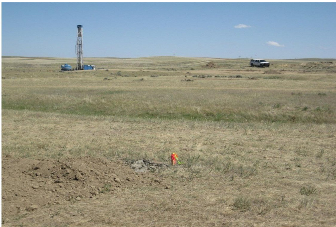
Figure 10.1. Drilling rig and logging truck from completed location on Southwest Reno Creek Unit
