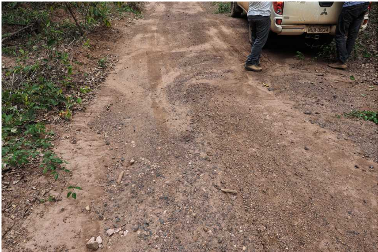
Photo 1 Serra Morena Project: Clasts in roadbed
