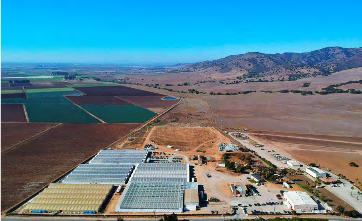
Retrofitted Canopy Currently Operational
