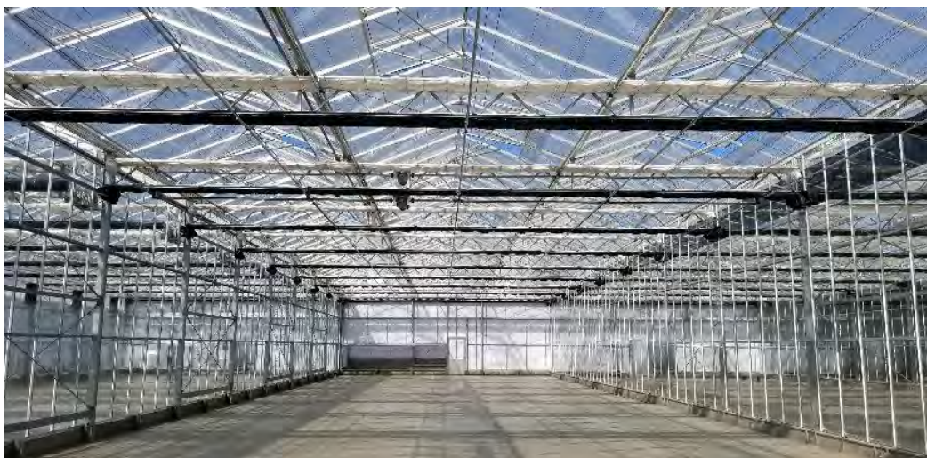
Greenhouse 1 under construction
