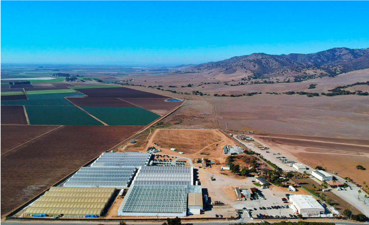
Retrofitted Canopy Currently Operational
