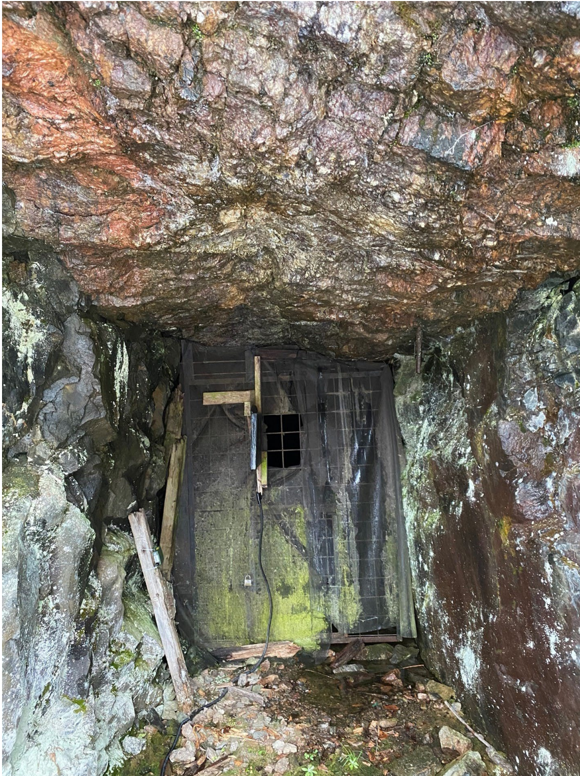
Figure 12-6: Richard Lake Property west upper adit entrance
