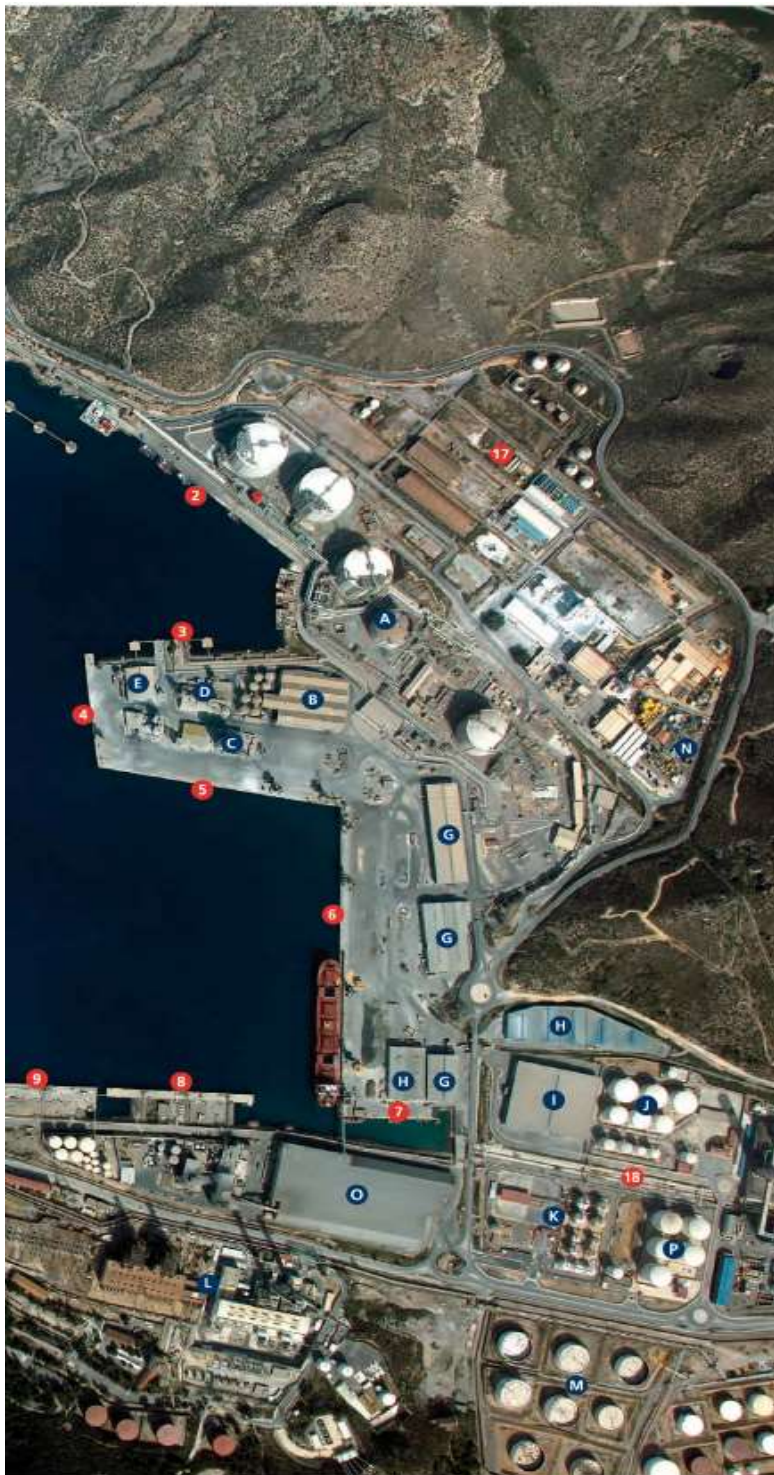
Figure 5.6: Port of Cartagena Surface Facilities
