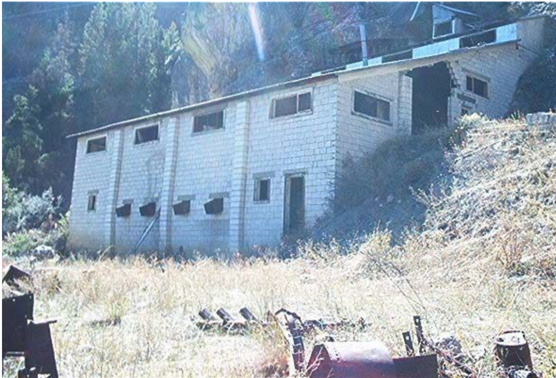
Figure 4-3 Twin Peaks Mine Mill Building in 2006
