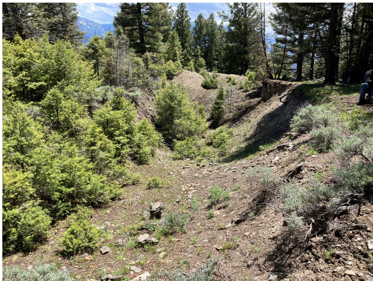
Figure 16-2 Dozer Cut Copper Prospect 1 km North of Twin Peaks Mine
