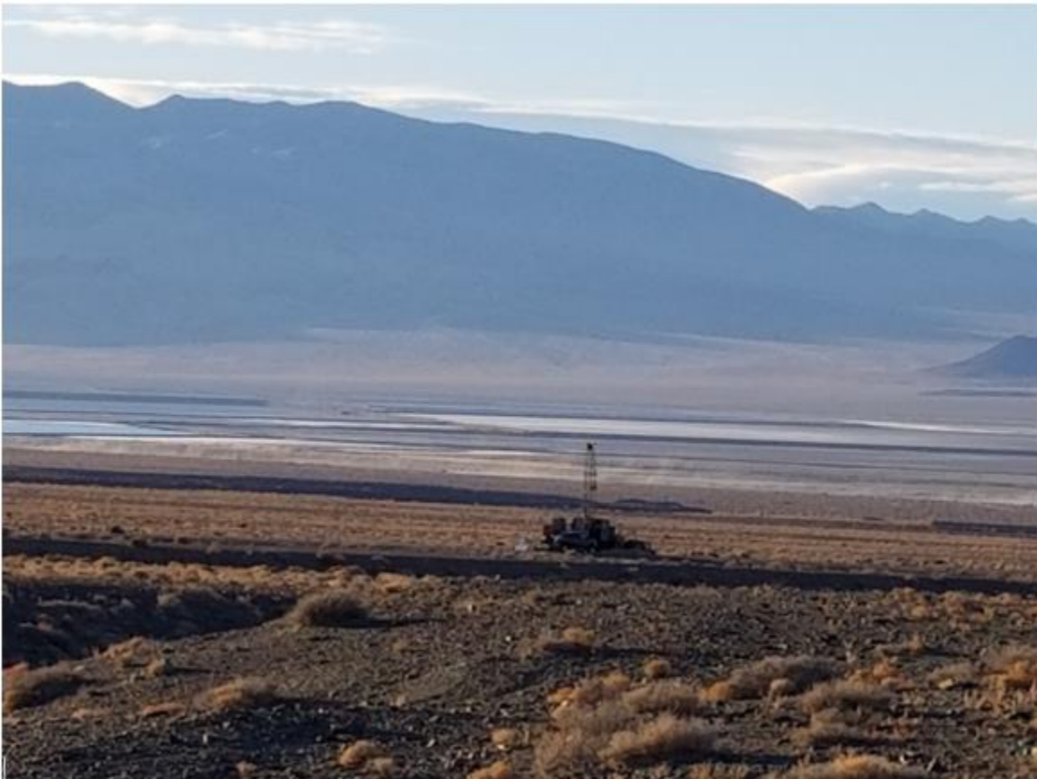
Figure 2 – Noram drill rig operating at Site A (CVZ-63) on the northeastern extent of the Zeus Property. Albemarle’s Silver Peak lithium brine evaporation ponds visible in the background
