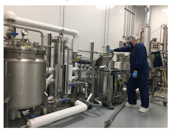
Figure 1 - Cryo-Ethanol Extraction System Installed in Adastra
