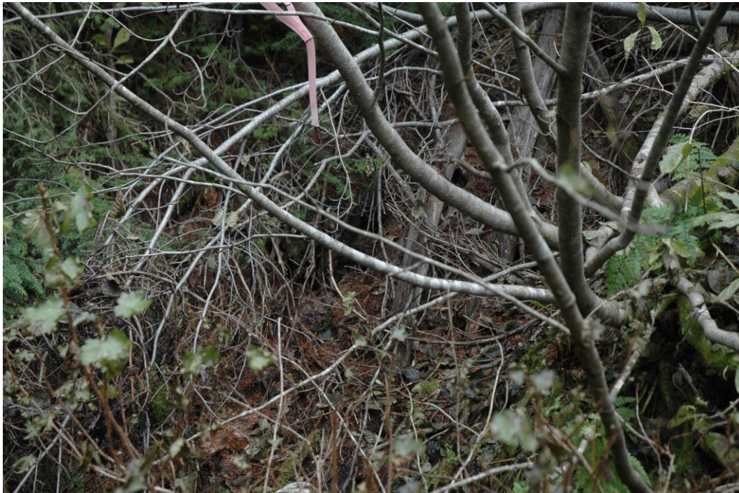
Photo 31 Caved entrance of the Gibson Adit 1
