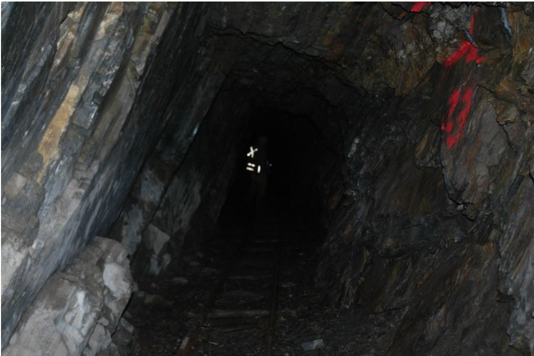
Photo 36 The Lower Adit Following Bedding and the Bedding-Parallel Mineralized Band in Top Right Corner
