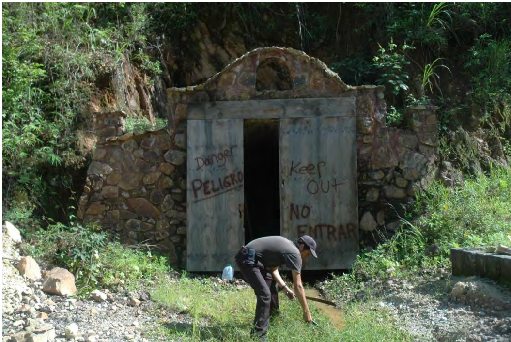
Plate 13: Entrance to the La Mina California mine.
