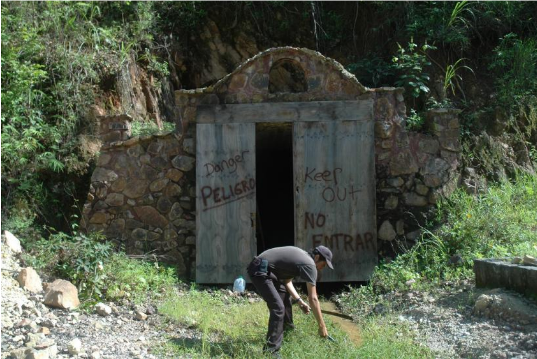
Photo 14 Entrance to La Mina California
