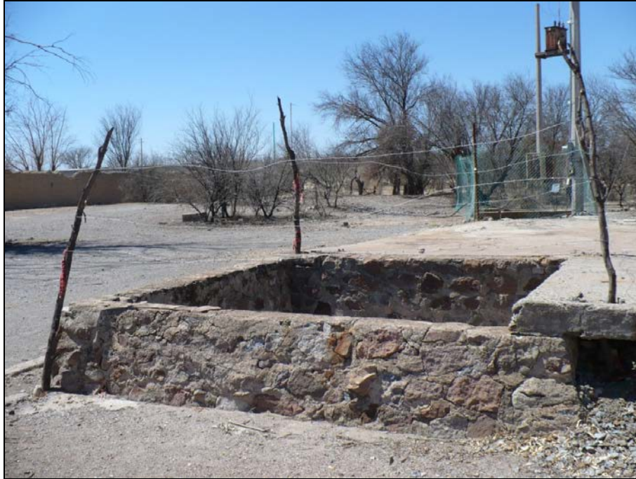
Figure 12-3: Water well at logging compound
